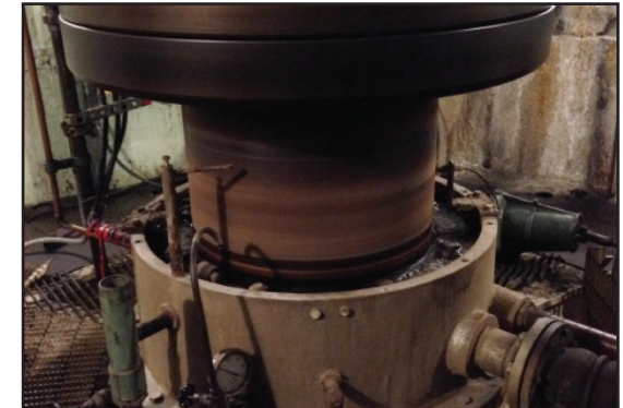
The station experienced increased uptime and saved over $33,000.
